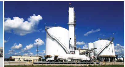
Linweld Air Separation Plant - Waverly, NE
