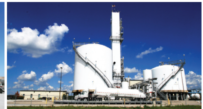
Linweld Air Separation Plant - Waverly, NE
