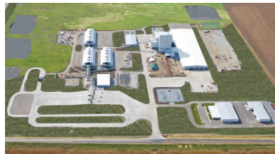
Monsanto Production Facility - Waco, NE
