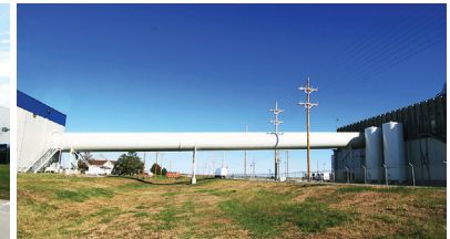
Excel Connecting Tunnel - Schuyler, NE
