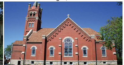
Saint Joseph's Catholic Church Auburn, NE
