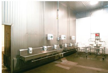
Plumbing and Electrical Modifications
