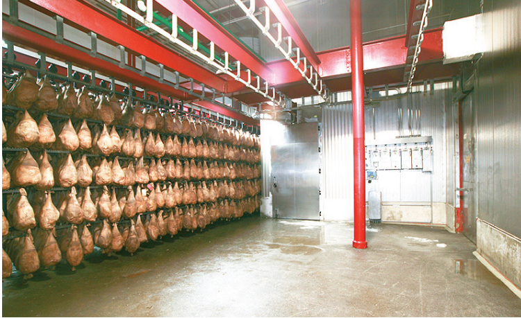
New Blast Freezer Door and Hardware
