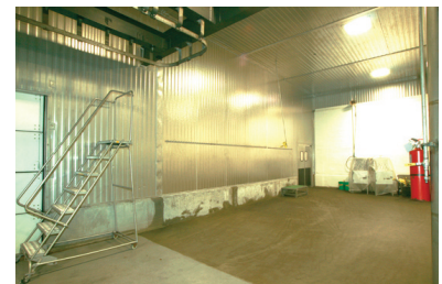
New Cast-in-Place Concrete Stem Walls and Wall Panel Installation
