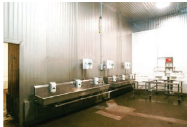
Plumbing and Electrical Modifications
