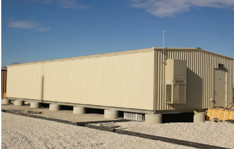
Typical Installation - Electrical Substation; Topeka, Kansas
